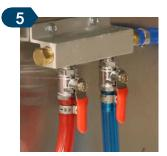
Turn the gas shut-off valve to the "**ON/DOWN**" position.
