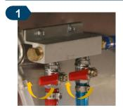
Start with the gas shut-off valves in the "OFF/UP" position *and* with the valve on the gas tank fully open
